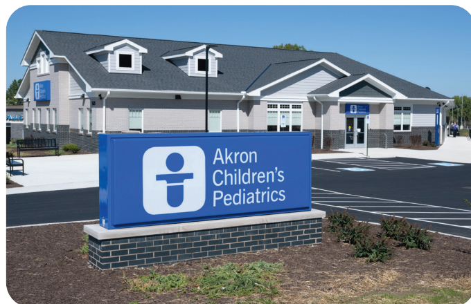
The new Akron Children's Pediatrics office brings high-quality care closer to families in and around Cuyahoga Falls.
